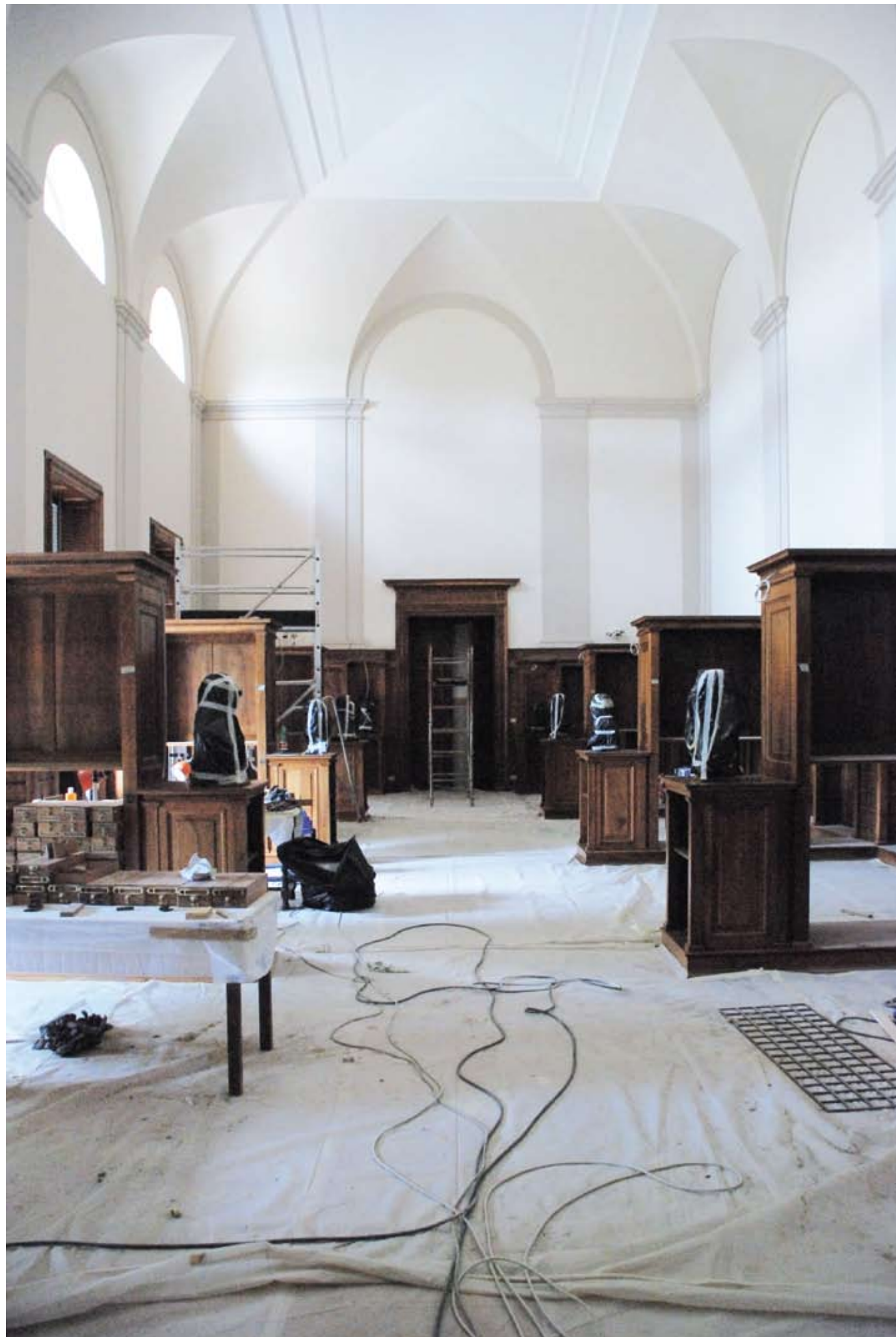
Arthur Ross Reading room site preparation.
